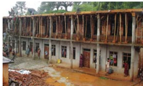
Bhubaneshwori school, under construction
