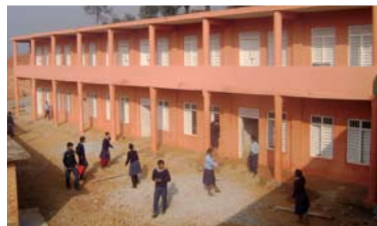
Bhubaneshwori school, after
