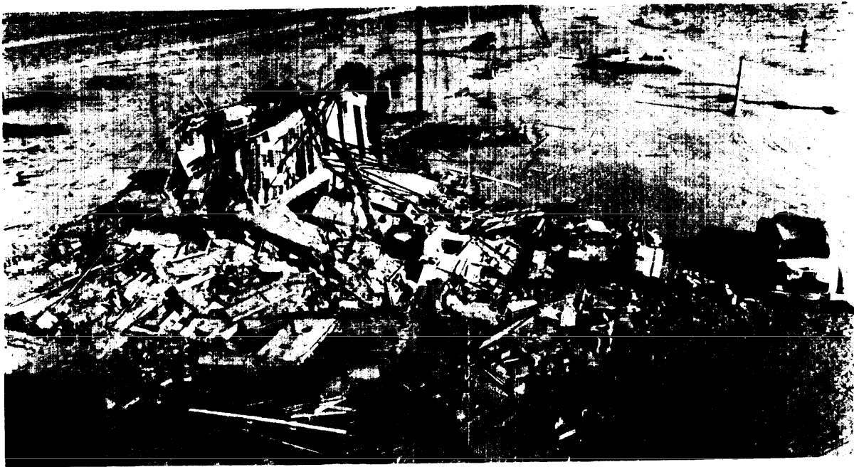
Damage to unreinforced brick house (5-psi overpressure)
