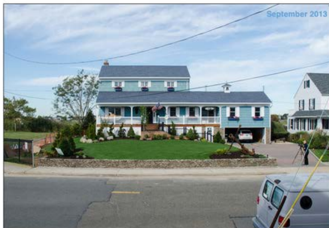
After the surge from Hurricane Sandy flooded their home with 5 feet of water, these homeowners elevated their house to mitigate against future disasters.
