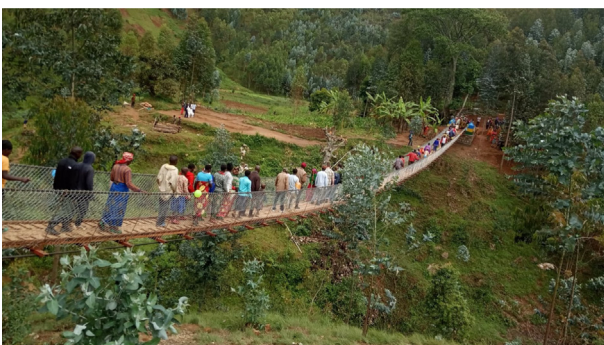
Fig. 1. An example Bridges to Prosperity trailbridge in Rwanda (Credit: Envision Photography/Bridges to Prosperity).
