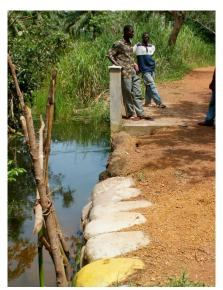
The side-walls of the culverts are a waste of cement (see photos), as they have no load bearing function. Marking the position of the bridge could be done with sticks or brick pillars.
