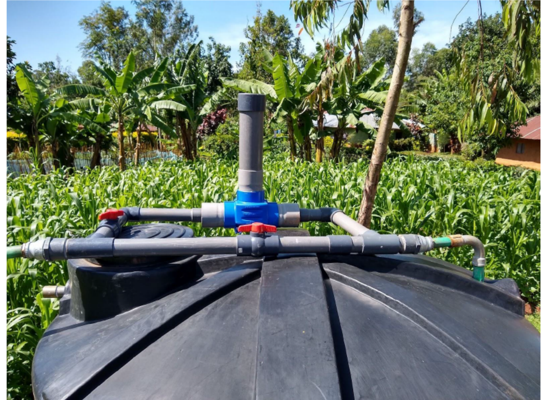
In-line chlorine dispenser. Source: Evidence Action.
