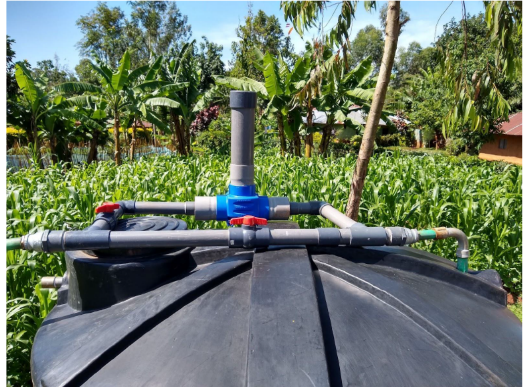
In-line chlorine dispenser. Source: Evidence Action.
