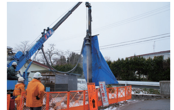
Wells under construction
