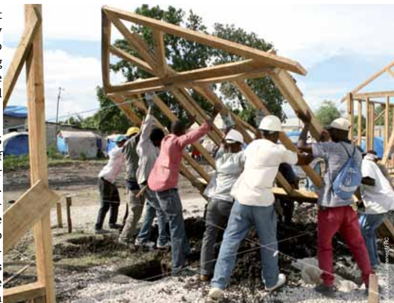
Workers and Red Cross Red Crescent carpenters erect a transitional shelter in l'Annexe de la Mairie, Port-au-Prince.
