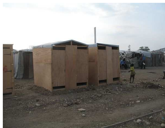
Sanitation is a major issue in addressing the needs of earthquake affected communities. The challenge posed is that Port-au-Prince is an urban area and much of the ground is either paved or difficult to drill through. Example of temporary latrine with underground tanks. Source: Hope Weiner / IFRC
