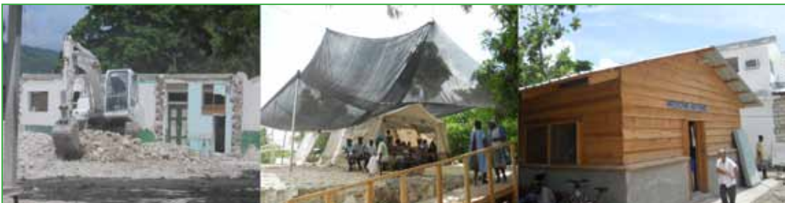
St. Michel Hospital in Jacmel suffered heavy damage during the earthquake. Some portions were demolished and new wings have been erected.
